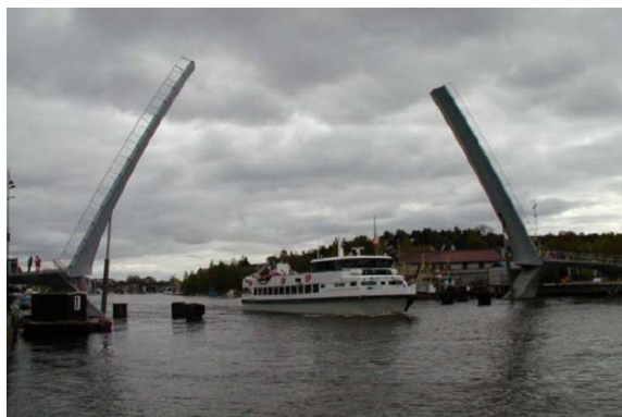
Figure 6: Balance Bridge for pedestrians in Fredrikstat, Norway
